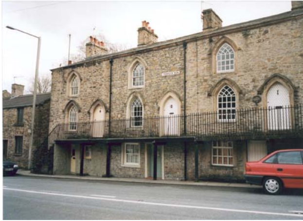
Terrace Row in Whalley Road have attractive Gothic details
