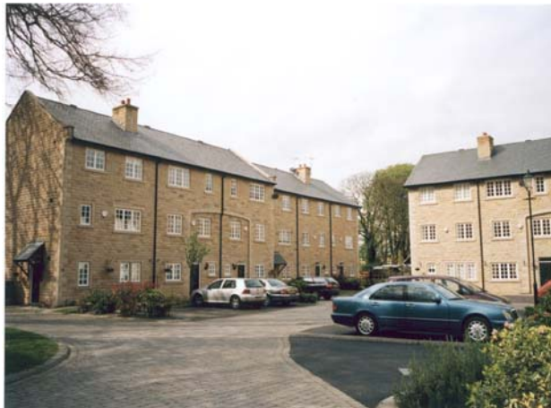
Modern development : Corn Mill Mews, off King Street
