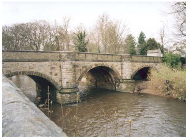
Whalley Bridge, over the river Don, from the south-east side
