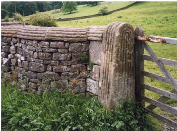
Stone gate pier and wall coping with characteristic pattern of incised lines
