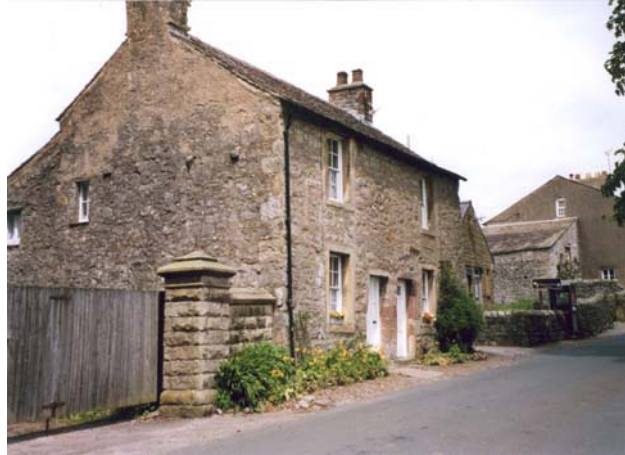
Nos. 22 and 24 Church Street
