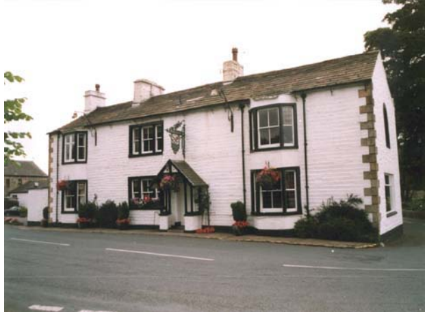
The Spread Eagle, with its watershot stone façade
