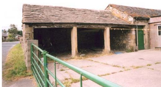
Southport House, cartsheds
