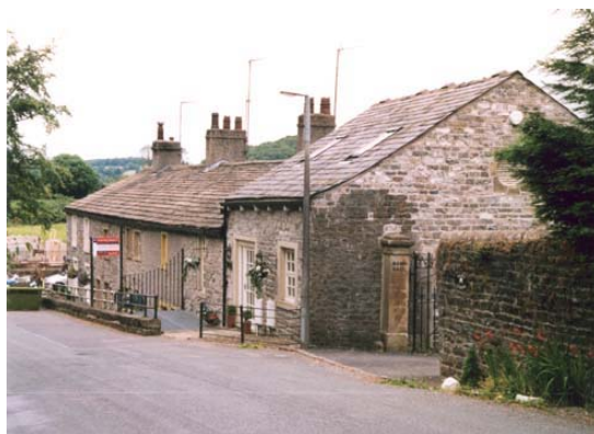
Bank Hall Cottages
