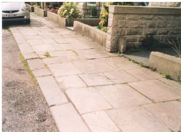
Stone paving in Pendle Street West
