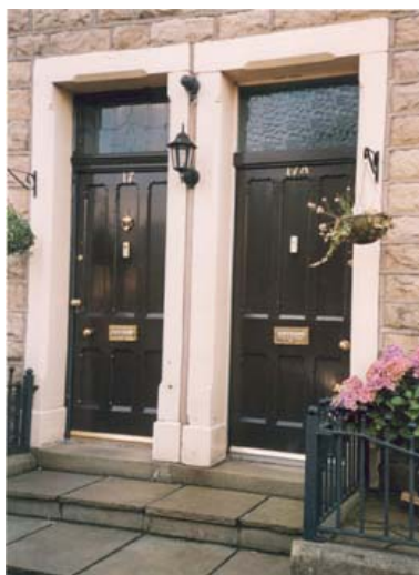
Original timber doors in Pendle Street East
