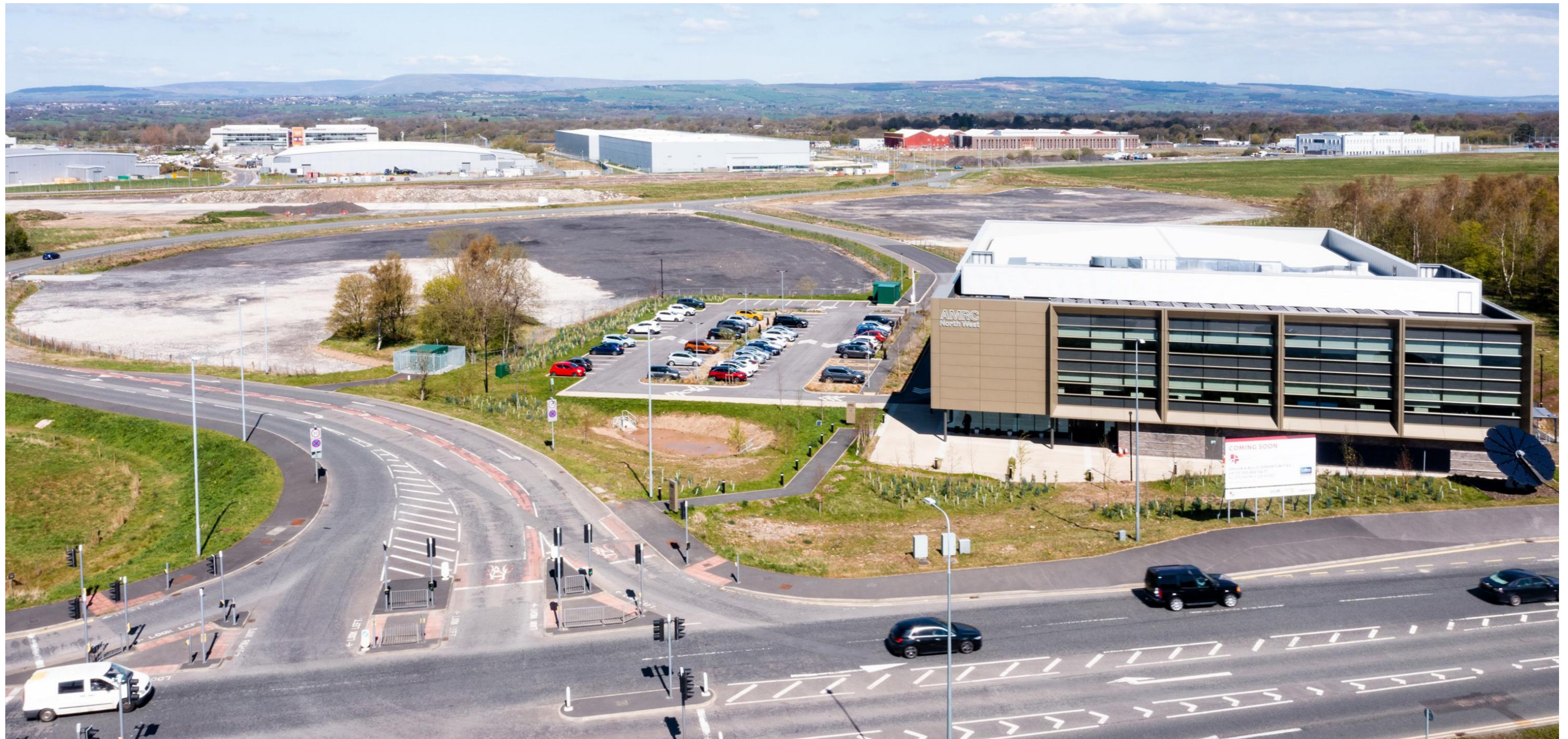
Fig. 9 - Existing aerial view of the Samlesbury site.
