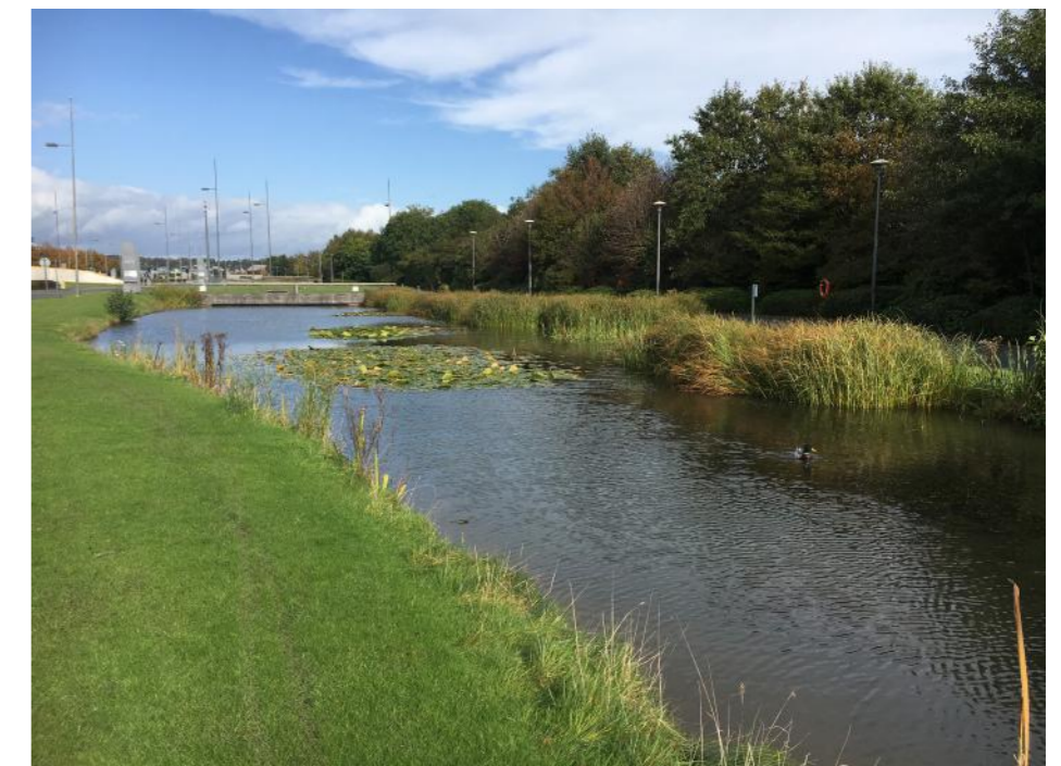
Fig.27 - Example of a Sustainable Urban Drainage System.
