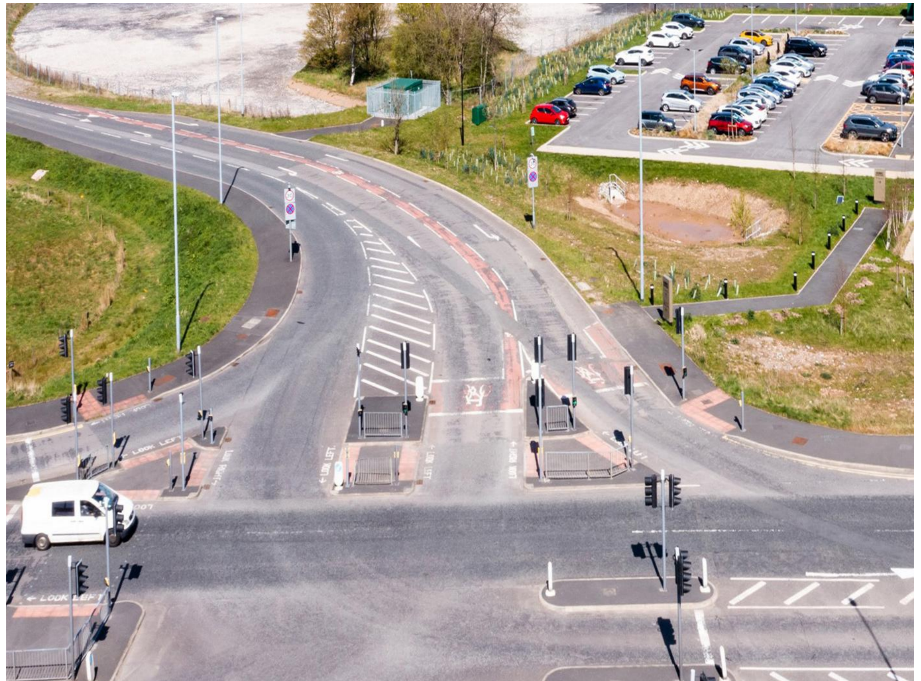
Fig. 34 - Existing photograph of the A677 junction.
