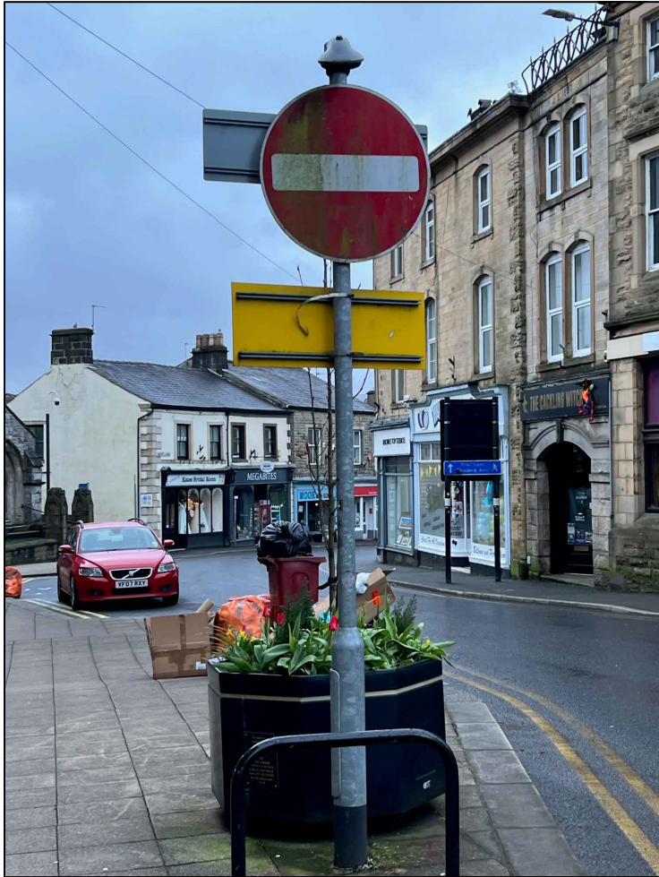
SIGN LOCATED ON NORTH SIDE OF CASTLE GATE, FACING PARSON LANE
