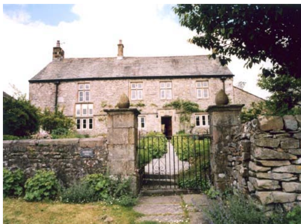
Grade-II listed Salisbury Hall Farm
