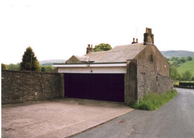
Poorly sited garage at the rear of Newton Hall
