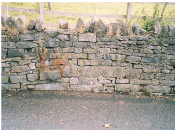
Stone walls are typical of the area
