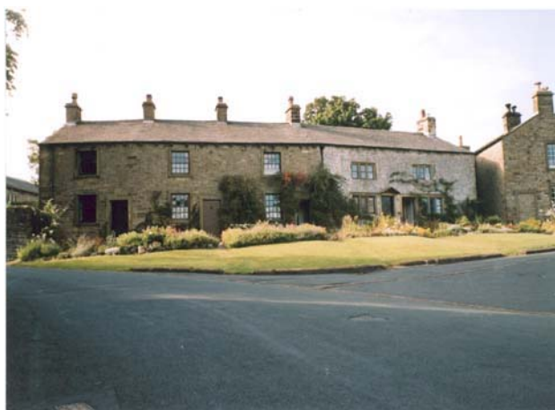
Nos. 2 – 6 Main Street overlook the open space east of the churchyard
