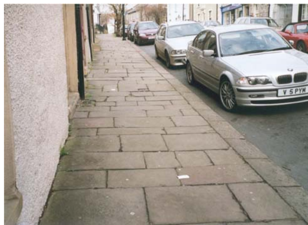
Natural stone paving, Church Street is a remnant of Clitheroe's historic floorscape
