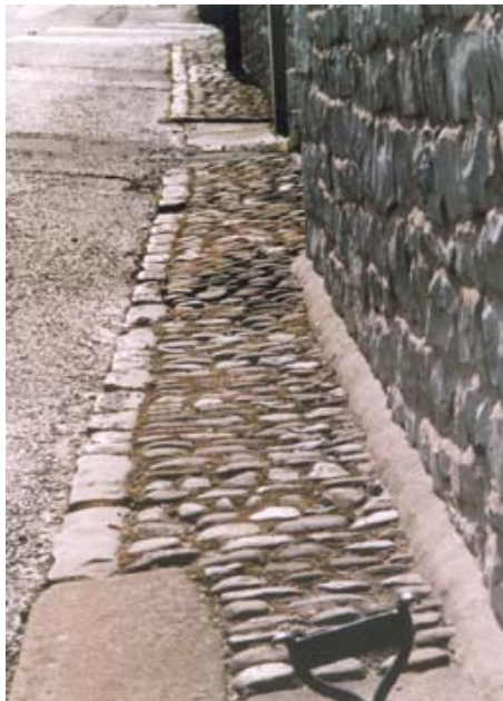
Historic paving in beside No. 1 Ribble Lane
