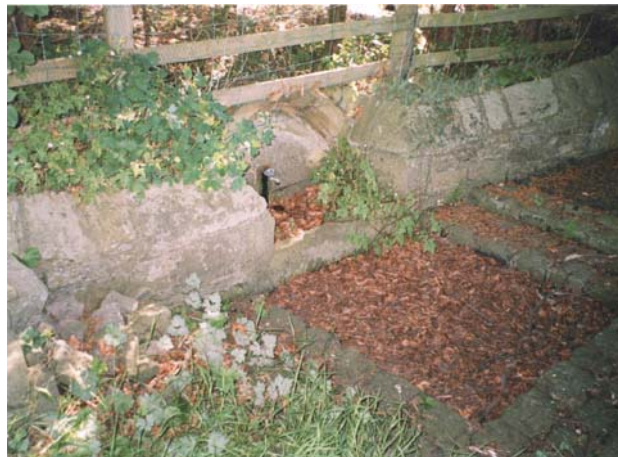
Site of old spring beside Stocks House
