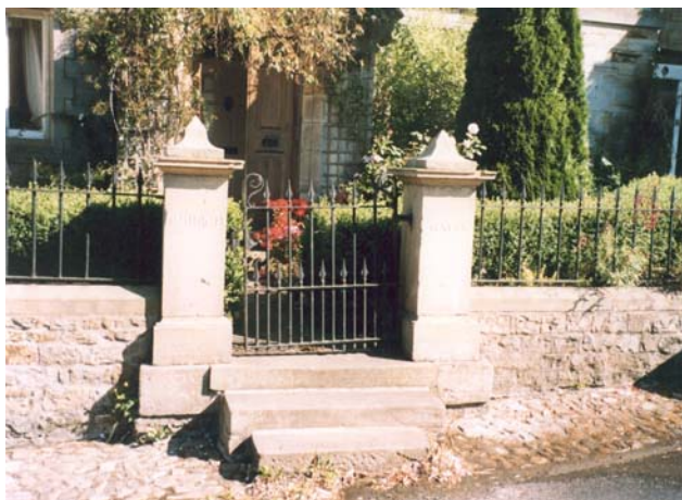
Ornate gate piers and old iron gate at Church Gates, Gisburn Road
