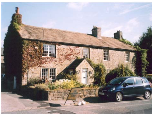
Local stone is the prevalent building material
