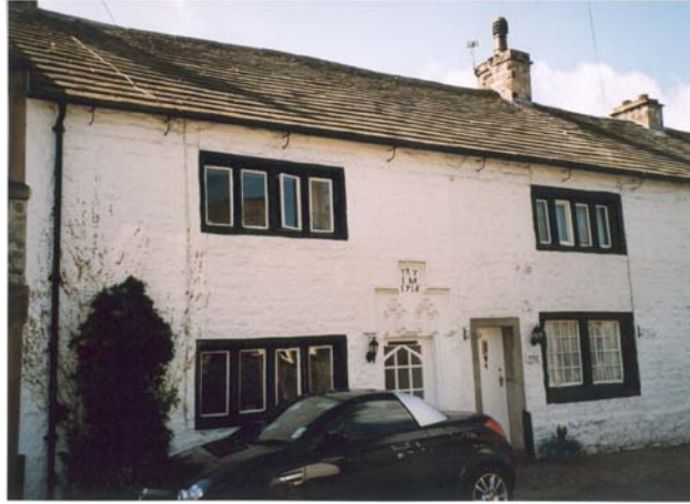
No. 4 Main Street, an 18 th century house with stone roof tiles
