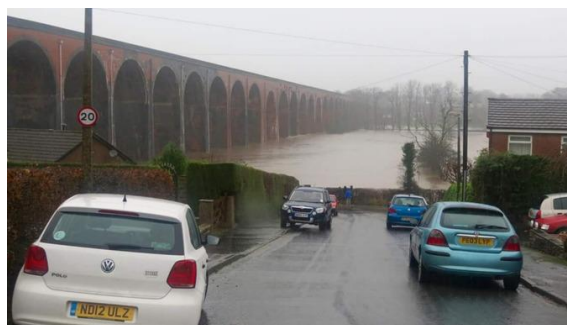
River Calder at Billington - Whalley Viaduct
