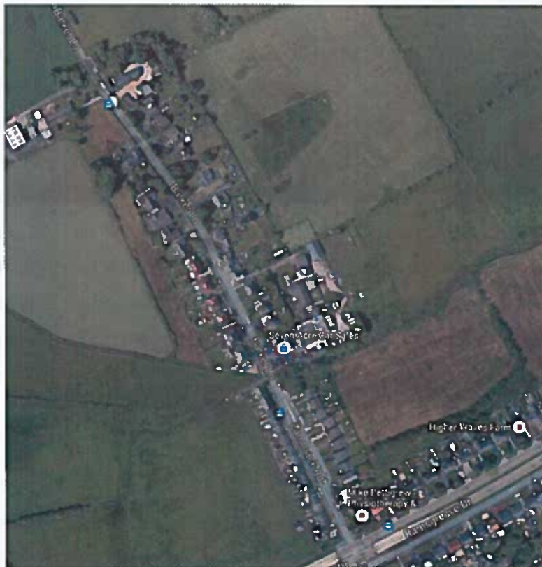
Figure 1 – Aerial view of development on Barker Lane
