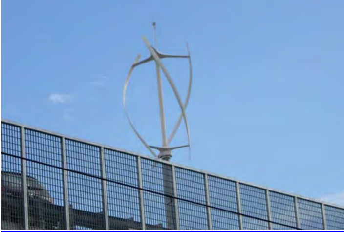
Wind Turbine at Preston Train Station
