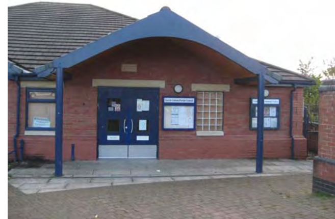
Community Centre at Cottam
