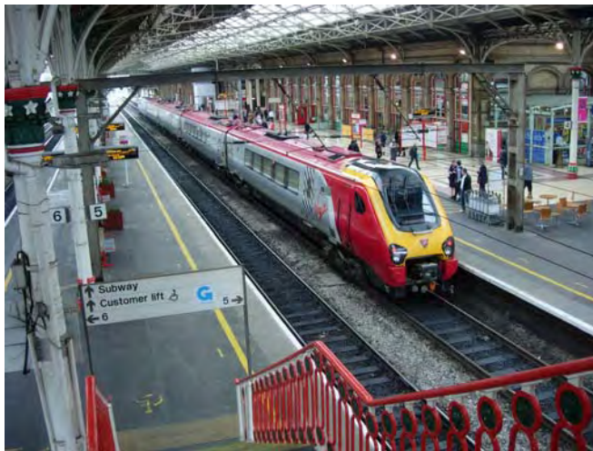
Preston Train Station
