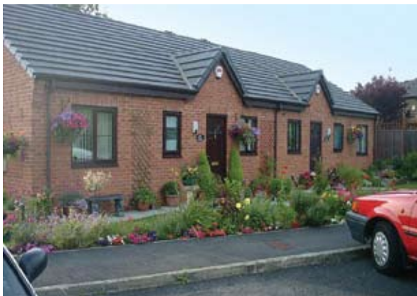
Showley Court LA owned sheltered accommodation, Ribble Valley
