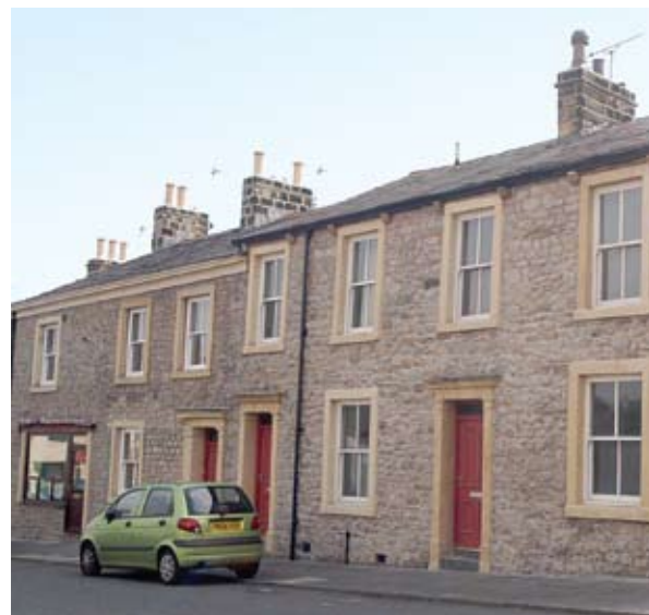
Landlord Renovation Grant - Group Repair Whalley Road, Ribblesdale
