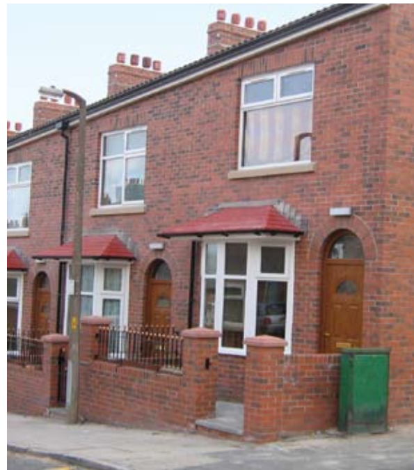
Group Repair After Cheetham Street Blackburn
