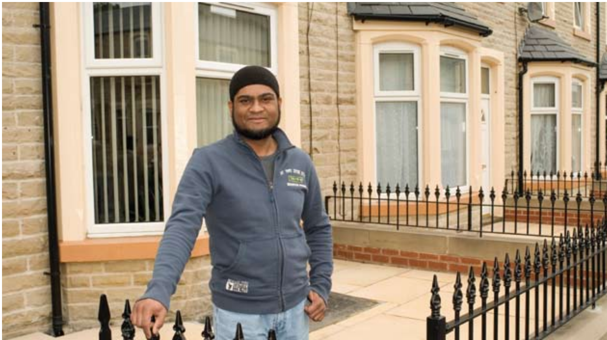
Improvement Scheme Colne Road, Brierfield
