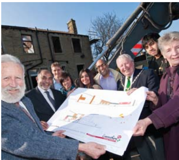
Starting work on the Bradley Youth Centre site, Nelson... a new flagship Youth Centre and supported housing scheme will be built here
