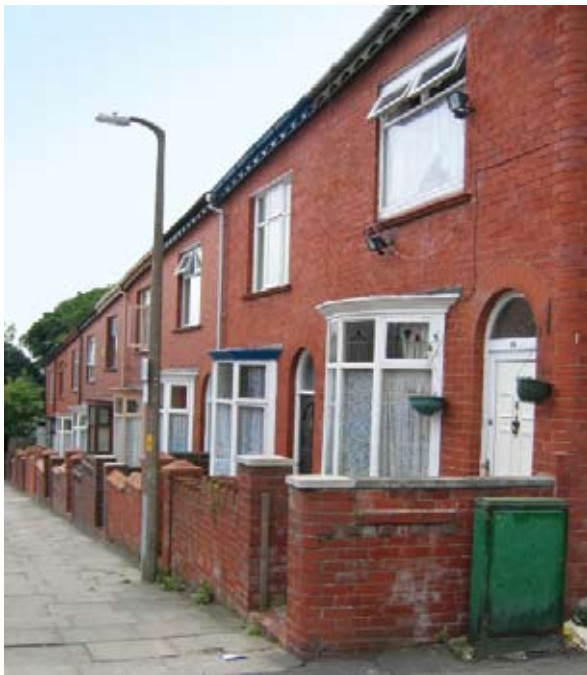
Group Repair Before Cheetham Street Blackburn
