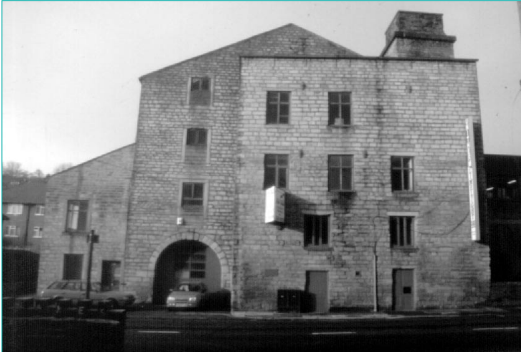
Photo 8. Textile Mill, Rossendale
