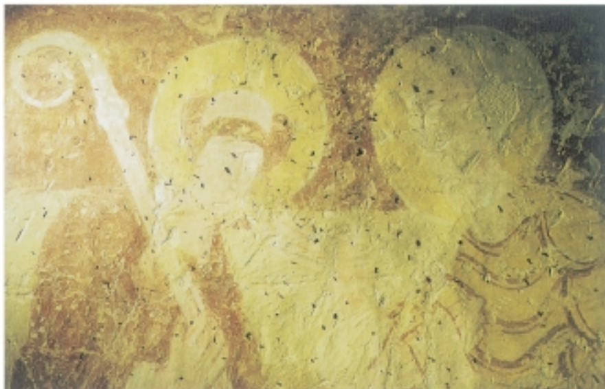
The internationally renowned scheme of wall paintings (dated c 1100) at Clayton Church, East Sussex, has been exposed to bat excreta as the result of this church being used as a roosting site. While the presence of urine can often be difficult to see because of the porous nature of a wall surface, droppings are more easily identifiable, as seen here
