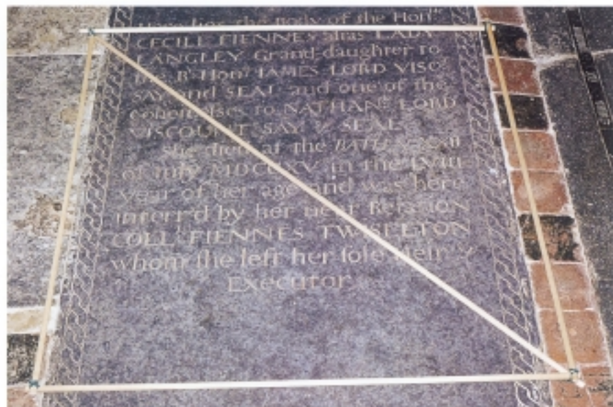
Since evidence for the presence of bats can be detected through damage to woodwork, stone, metals, and other vulnerable surfaces, it is useful to chart these effects by counting the visible damage marks on surfaces and plotting these on a plan of the church. A measuring frame, as shown here, assists in developing a systematic approach to this exercise. Such information will give a useful indication of both the rate and distribution pattern of bat excreta throughout the building
