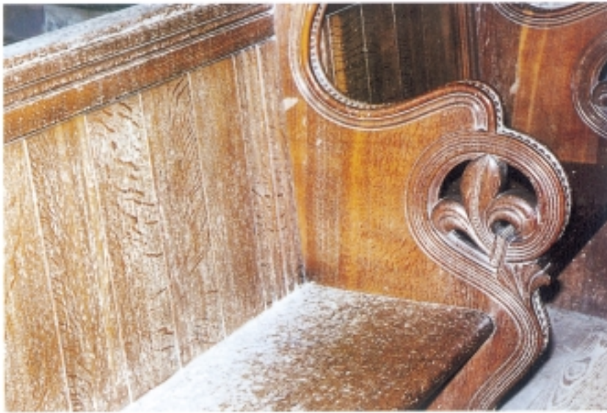
At Brinkburn Priory, Northumberland, a nineteenth-century pew displays evidence of both visual and surface damage to the wooden surface from the development of microbiological organisms forming on an area of extensive urine deposition
