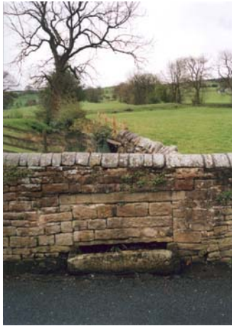
Walls, paddocks, springs and troughs are a feature of the village
